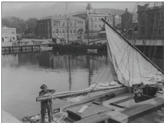
View across Constitution Dock to the Carnegie Building. Circa 1920.
